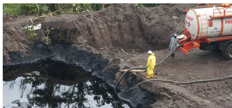
The heavy oil is being extracted and removed with tankers
