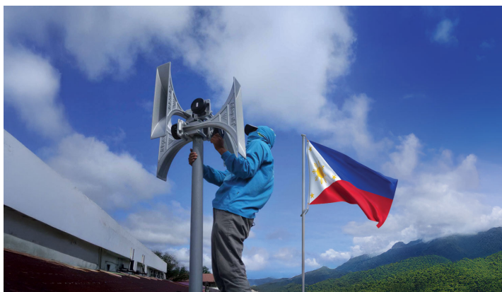
Person installing a electronic siren in the Philippines as part of a community early warning system.
