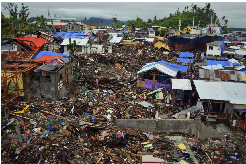
Severe destruction and damage in the aftermath of Super Typhoon Haiyan in Philippines
